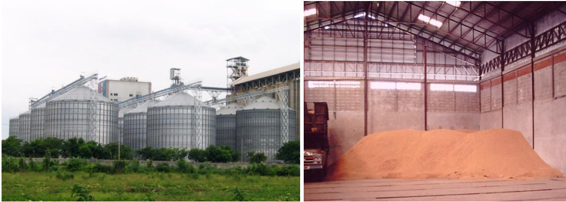
Figure 3: Steel silos are not commonly used in the tropics because of condensation problems with high moisture grains; few millers and traders have warehouses for bulk storage (right)
