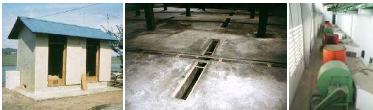
Figure 23: Korean low-temperature in-bin drying and storage system (IBDS) at farm level (left), aeration ducts in a large storage system (center), and blowers and heaters for an in store drying system with 4 batches (right).
